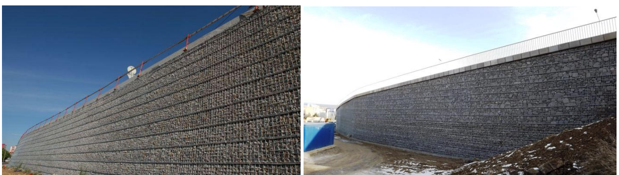
Boulder facing slope
